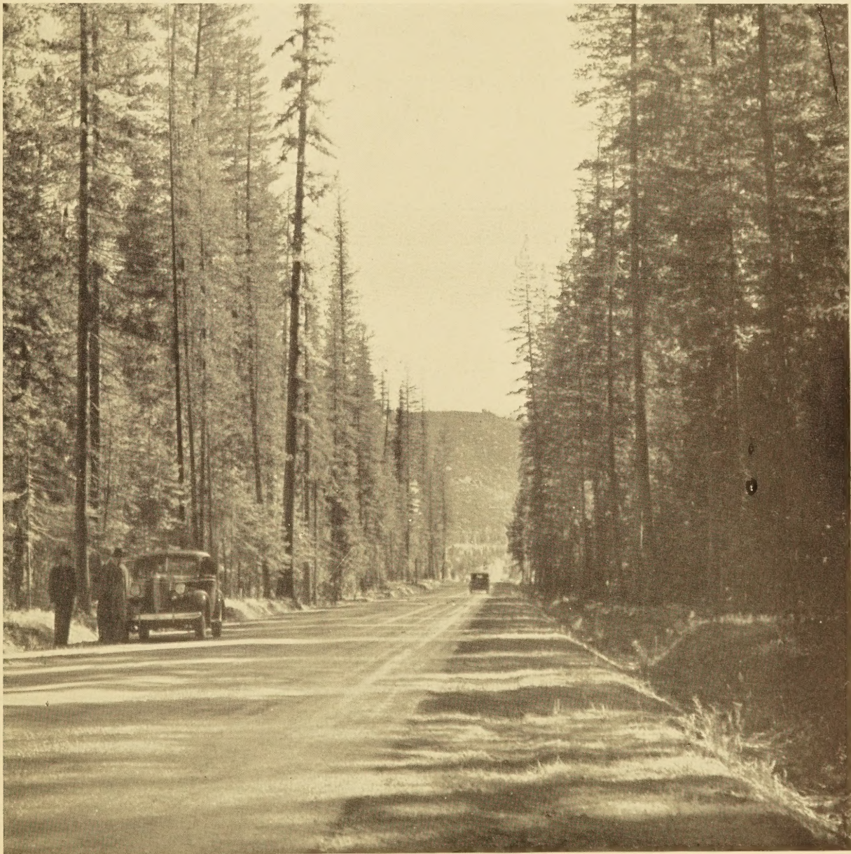
A SECTION OF U S 10 IN MONTANA
